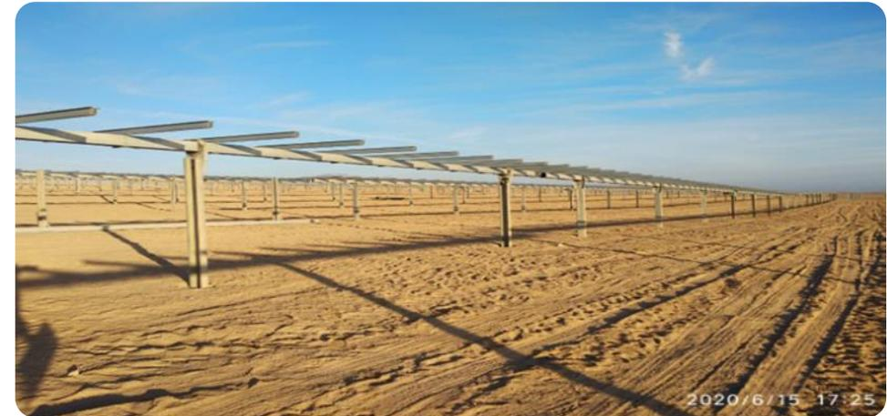
15.6k drill holes, 13k steel piles, 205 trackers, 11k solar modules assembled
