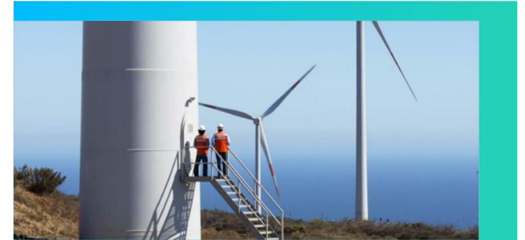
48 MW (24 Vestas V90 WTGs(\*), 80m hub height, 90m rotor diameter, 125m total height) 1,000 hectare site in Coquimbo region
