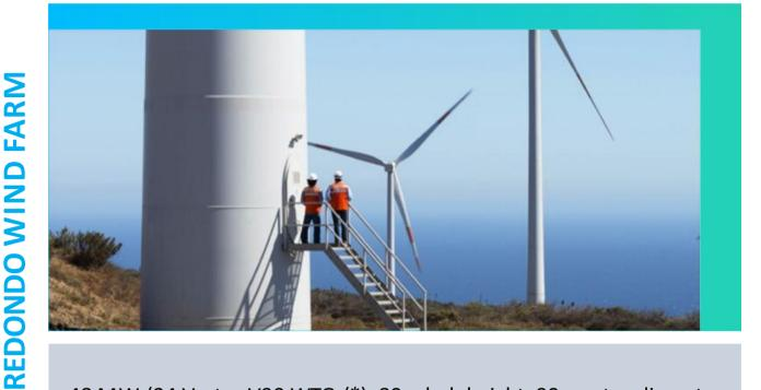
48 MW (24 Vestas V90 WTGs(\*), 80m hub height, 90m rotor diameter, 125m total height) 1,000 hectare site in Coquimbo region In operation since 4Q-2009
