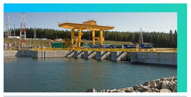
34MW run-of-river, 14Mm3 reservoir ~60km of Los Angeles, Bío-Bío. Operating since 2015. Powerhouse w/2 17.2MW Bulb-Kaplan units
