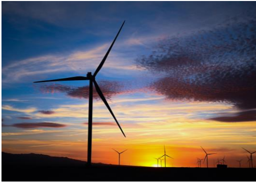
342MW Lomas de Taltal Wind US$468 million investment
