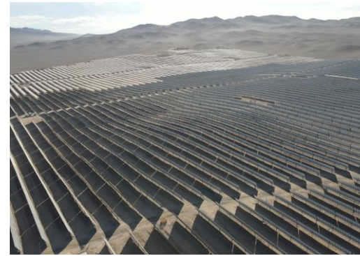
48MW / 254 MWh BESS Capricornio (storage) US$76 million investment
